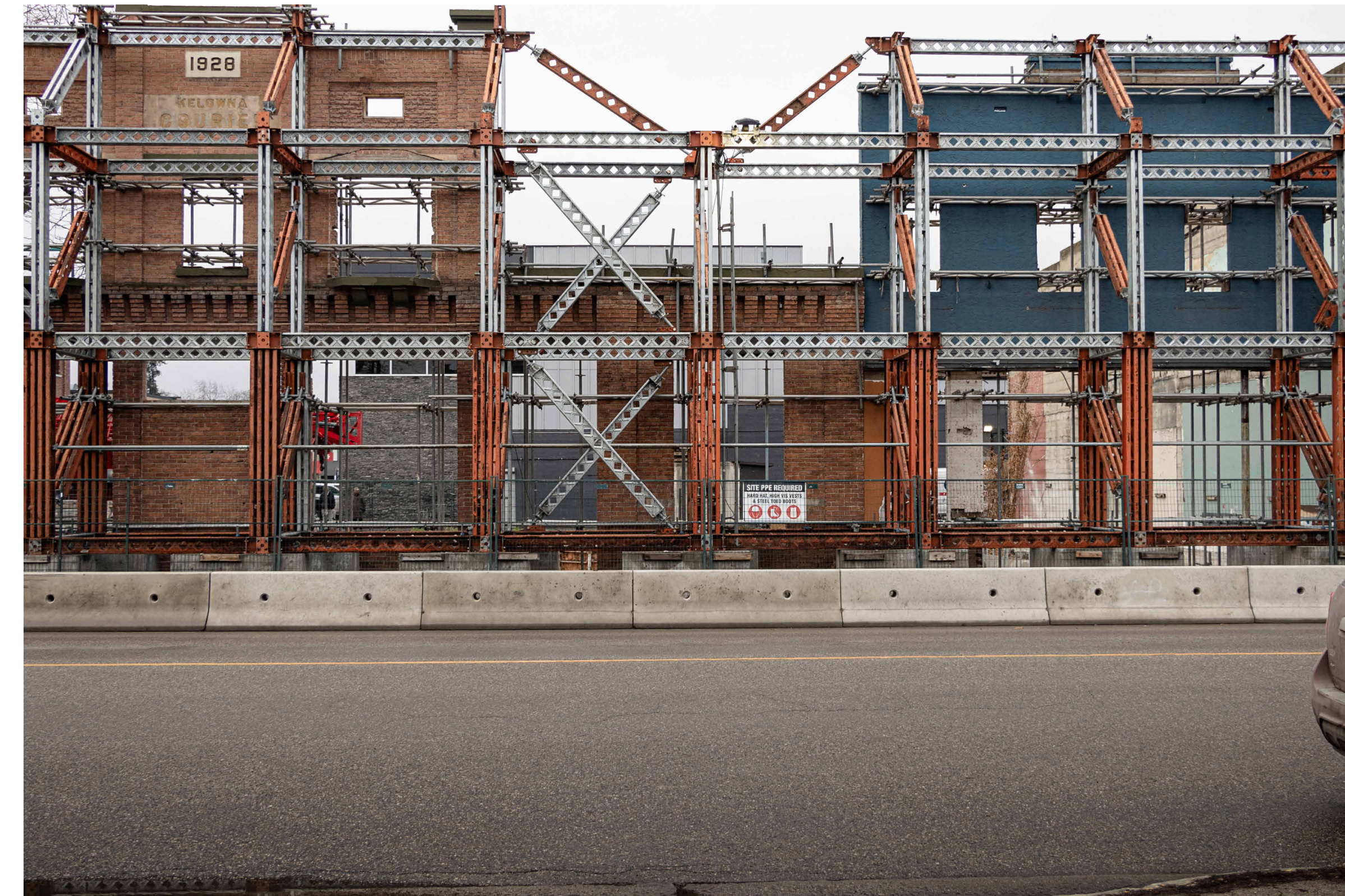
03/ EXISTING HISTORIC FACADE WITH TEMPORARY BRACING
